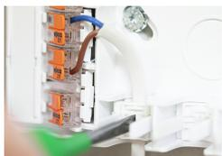
Insert the cable into the strain relief.
