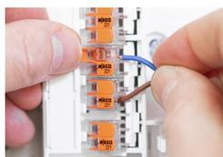
Inserting a conductor
