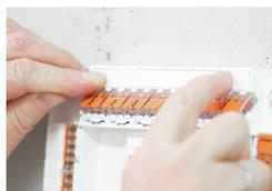
Snap the marking strips into the holder.
