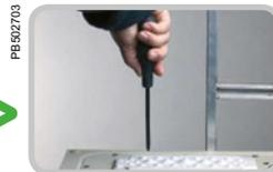
Make a small hole in the membrane.
