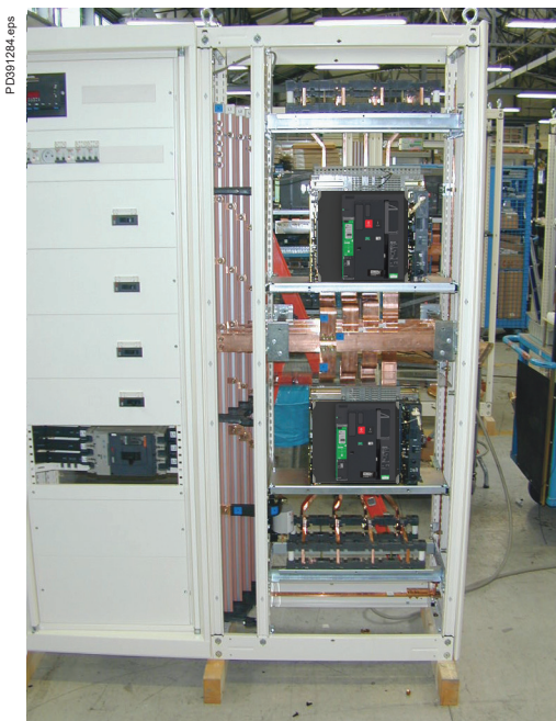
Source changeover system in 2 combined cubicles.
