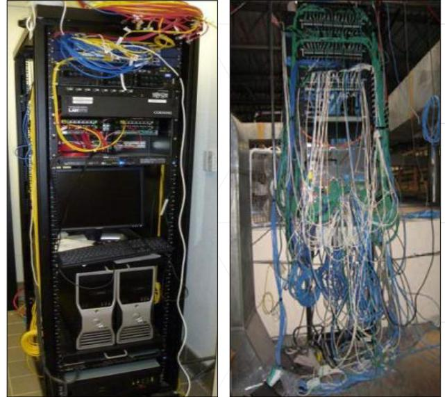
**Figure 2. Poor Industrial Network Installation Can Generate Unacceptable Downtime Risks**
