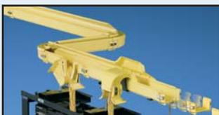
**Yellow** – Typical color used to denote a single mode fiber optic cable route.
