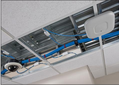
In today's enterprise, things are looking up ... literally. Look into that air-handling space above the ceiling tiles and you're likely to find wireless access points, security cameras, and connections for audio-video equipment, safety systems, and more.
