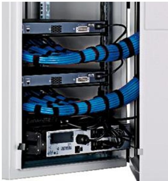
**Figure 13:** Copper-A (lower) and Copper-B (upper) copper cable bundles attached to strain relief bars.
