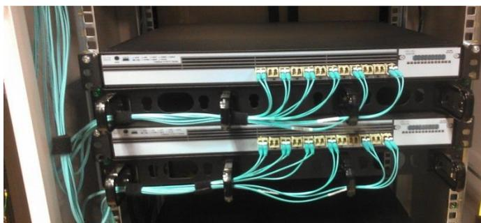
**Figure 21:** Fiber Switch A and B mounted to front rail showing fiber cable routing.
