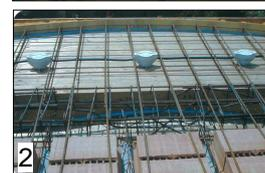
FISSARE LA CONTROCASSA ALL'ARMATURA NELLE POSIZIONI DESIDERATE (FIG.1) E POSIZIONARE I TUBI PER I CAVI DI ALIMENTAZIONE (FIG.2). FURTHER SECURE THE BOX TO THE REBARS IN THE DESIRED POSITIONS (FIG.1) AND PLACE THE CONDUITS FOR THE POWER CABLES (FIG.2).
