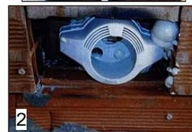
FISSARE CON SCHIUMA POLIURETANICA O MALTA CEMENTIZIA AD INDURIMENTO RAPIDO IN QUANTITÀ MINIMA E LASCIARE ASCIUGARE.
