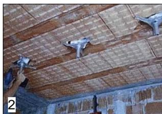
USING 3 TEMPORARY PLUGS IN THE APPROPRIATE SLOTS, OR WITH A SPRING-LOADED BRACE USED BY BRICKLAYERS, PLACE EVERYTHING ON THE ROUGH CEILING AND THUS KEEP THE BOX POSITIONED (FIG.1); THE CONFIGURATION OF THE SYSTEM ALLOWS THE BOX TO BE PRECISELY POSITIONED EXACTLY 1CM FROM THE BRICK, THUS LEAVING SPACE FOR THE SUBSEQUENT PLASTER. THE SIMULTANEOUS USE OF MULTIPLE APPLICATORS IS EASY (FIG.2).
