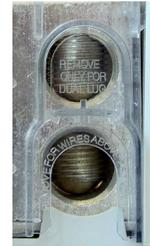
Standard dual lugs on 600A blocks and optional dual lugs on 400A blocks for easier wiring using two, smaller conductors.
