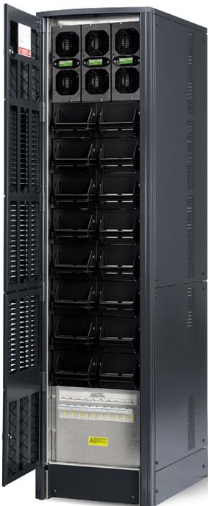
Trimod HE modular UPS with internal battery modules
