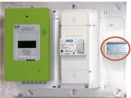
Up to 4 modules can be added to this electrical box, on the modular rail.
