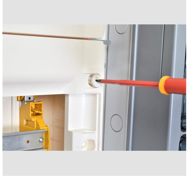
We recommend using a 6.5 mm flat screwdriver to open and close the XL<sup>3</sup> 125 cabinets, and also for positioning the faceplates with a ¼ turn, for which 1 nm tightening torque is sufficient.
