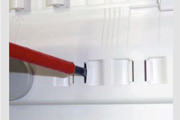
The cables or sleeves are then secured using Colring and Colson cable ties (up to 9 mm wide).
